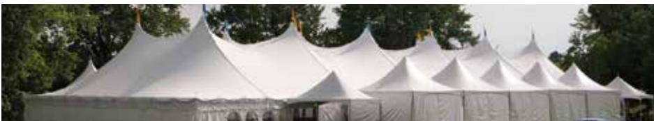
Polyplan Shield and Polyplan Tent Zero are lightweight and visually appealing membranes made by Sattler PRO-TEX. These high-quality coated fabrics come with a biocidal finish and an optional PVDF lacquer for best dirt repellency and durability.
